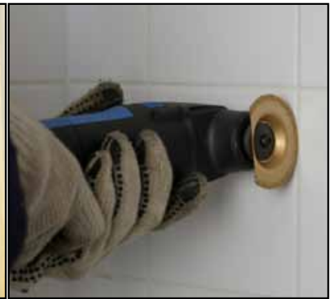
Demo of the grout removal head ideal for removing tiles.
